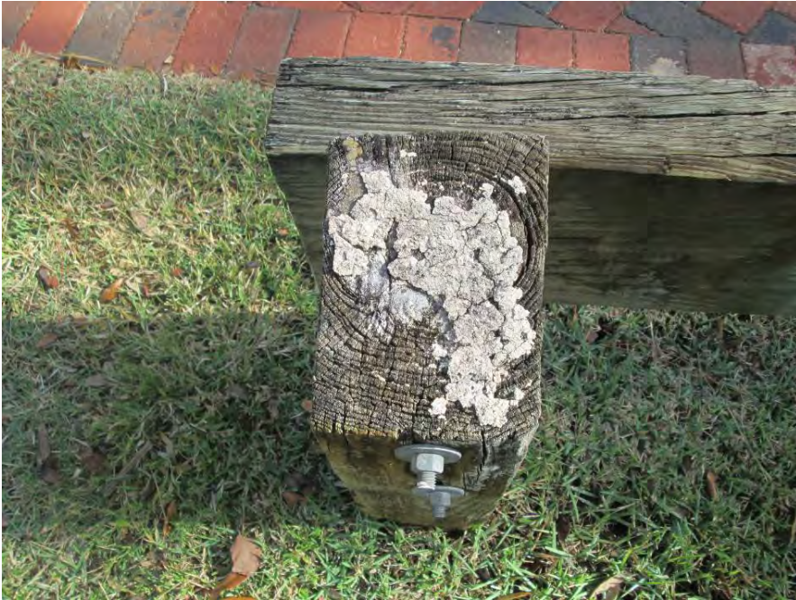
Sealant added to railing posts dried and cracked on Fish Hook Cove
