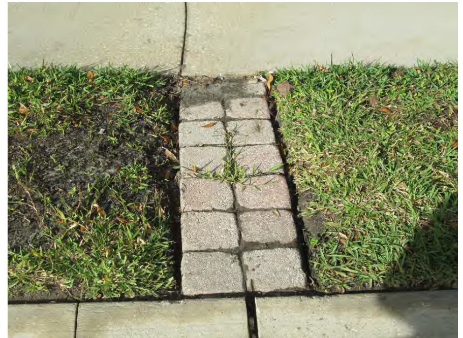
Brick sidewalk flumes on Winding Stream Way east of Rainbow Ct
