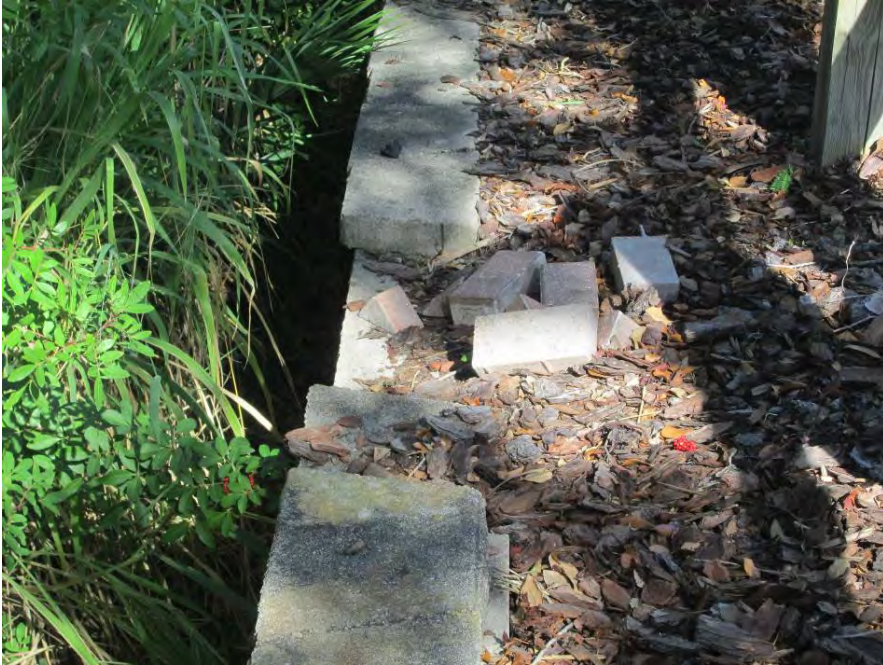
Top caps to Retaining Wall missing and brick debris along Discovery Terr
