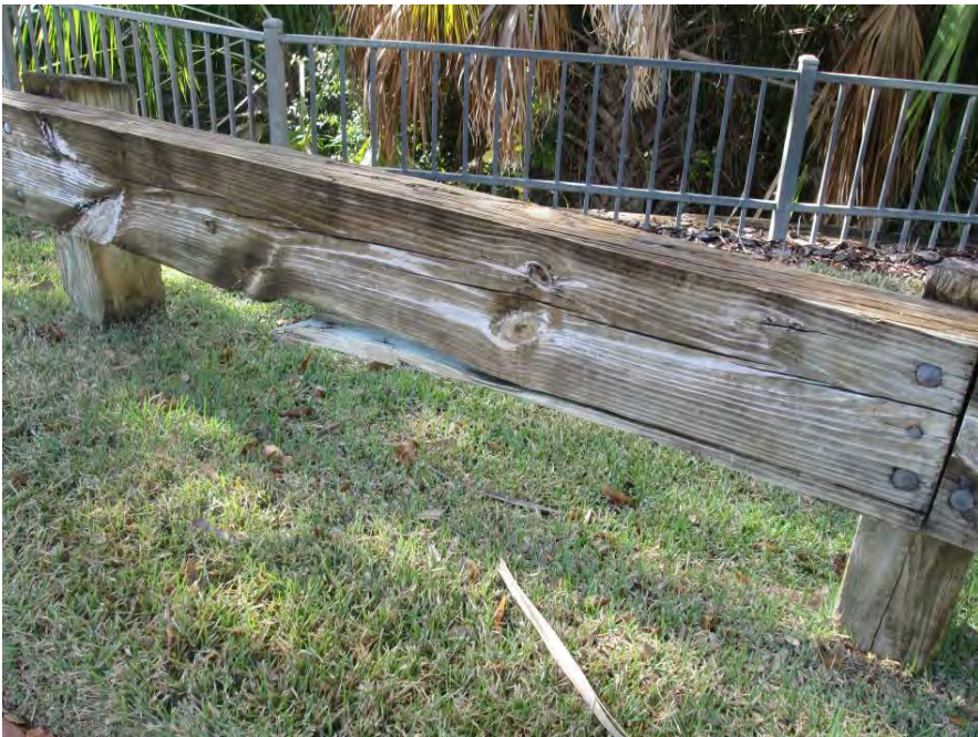
Railing splintering near Fish Hook Cove cul-de-sac
