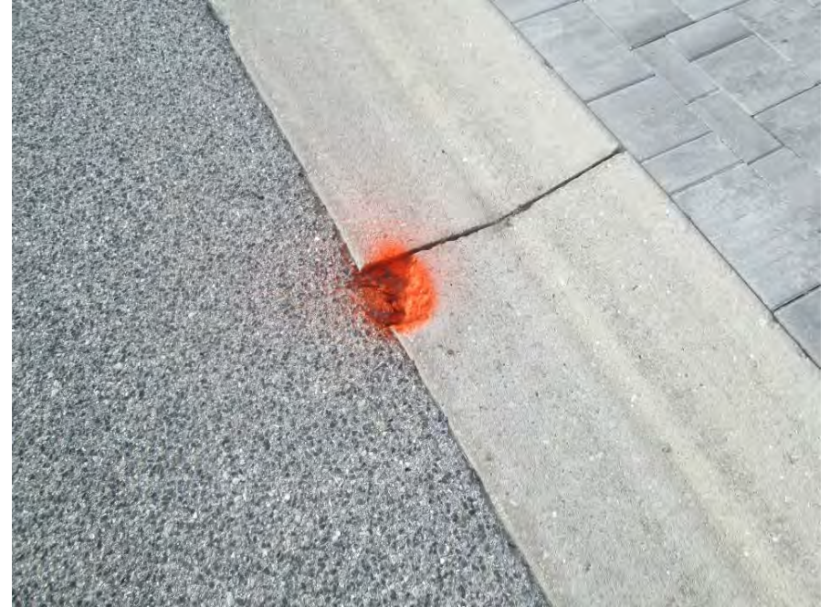
Winding Stream Way Lot 5, add epoxy grout
