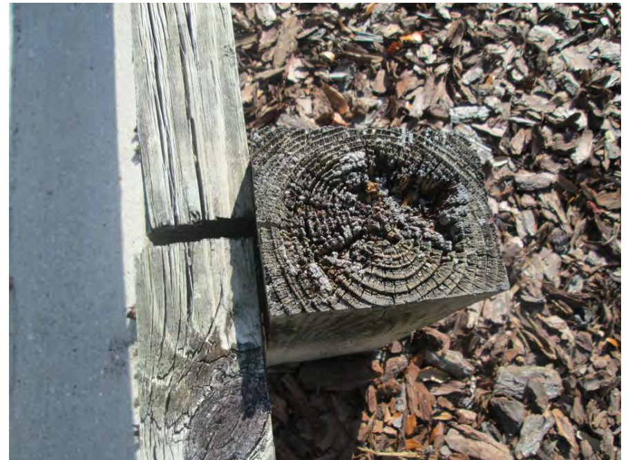
Add sealant to railing posts along Fish Hook Cove
