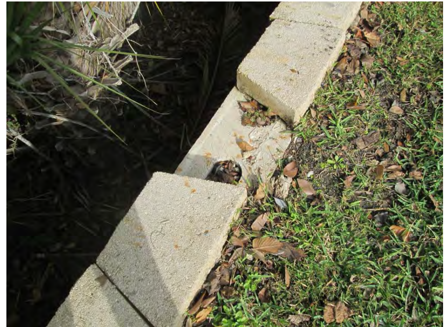
Top cap missing and loose on Retaining Wall north of Guard House
