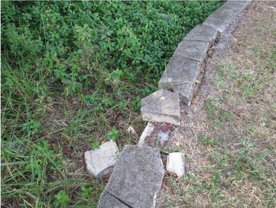
Top caps missing and loose on Retaining Wall on Conch Shell Terr
