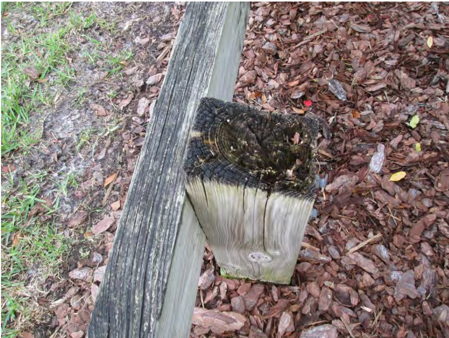
Add sealant to railing posts at Circle (Waterlefe Blvd/Winding Stream)
