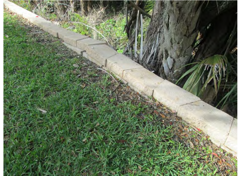
Top caps loose, north side Waterlefe Blvd Retaining Wall near Hole 5 Tee
