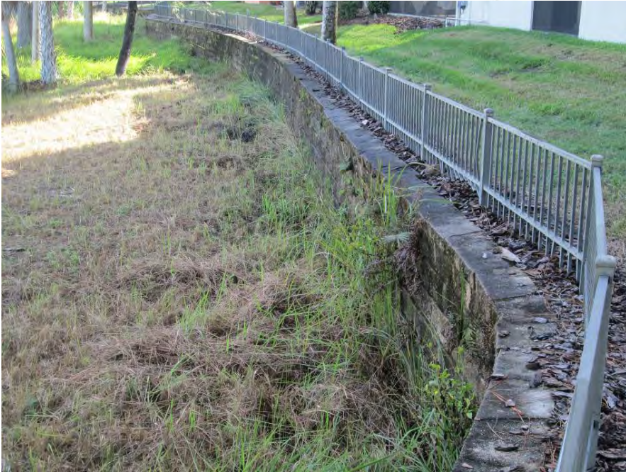
Spray vegetation on Fish Hook Cove Retaining Wall behind condos
