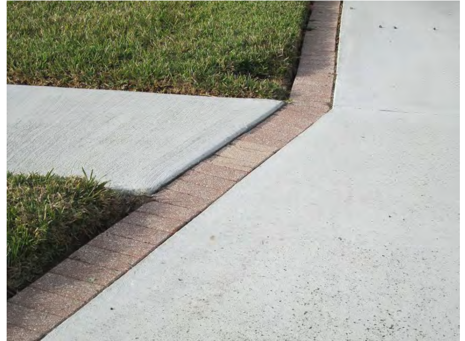
Settled Brick Pavers at driveway on Winding Stream Way (resident issue)
