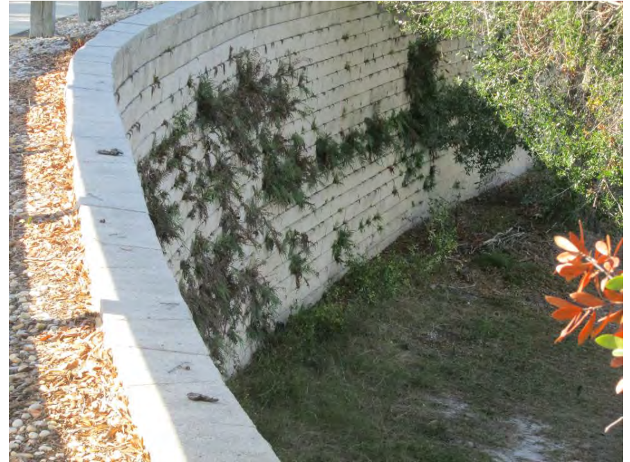
Spray vegetation on Retaining Wall at south end of Aqua Range
